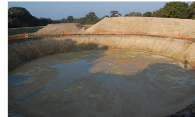
Excavation (Photo : VALOREM)
